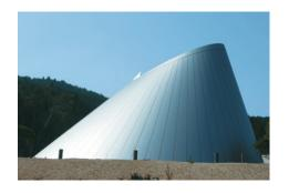
18.5 meters in length, the design drawn up by a world-famous architect required us to create plates more than three times the standard size. Through the application of our cutting facilities and surface finish ingenuity, we took on the challenge of implementing rounded-edge cuts, and succeeded in realizing the architect's original vision down to every detail.
