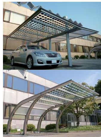
Car port with PV system Light through PV system which is unified with the roof.
