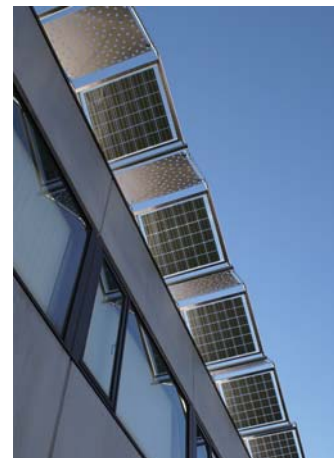
Canopy with PV system We arranged designed punching panels to the north.
