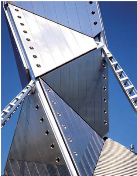
Built in 1990, the tower was a cutting-edge project in terms of its design, use of titanium and implementation.
