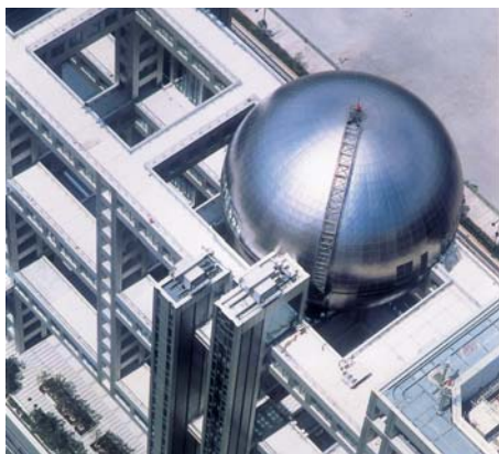
The 1,350 ton titanium observation sphere was an engineering marvel at the time.
