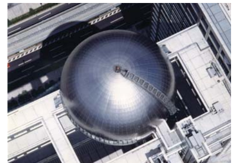
Raising the sphere into place was a major challenge.
