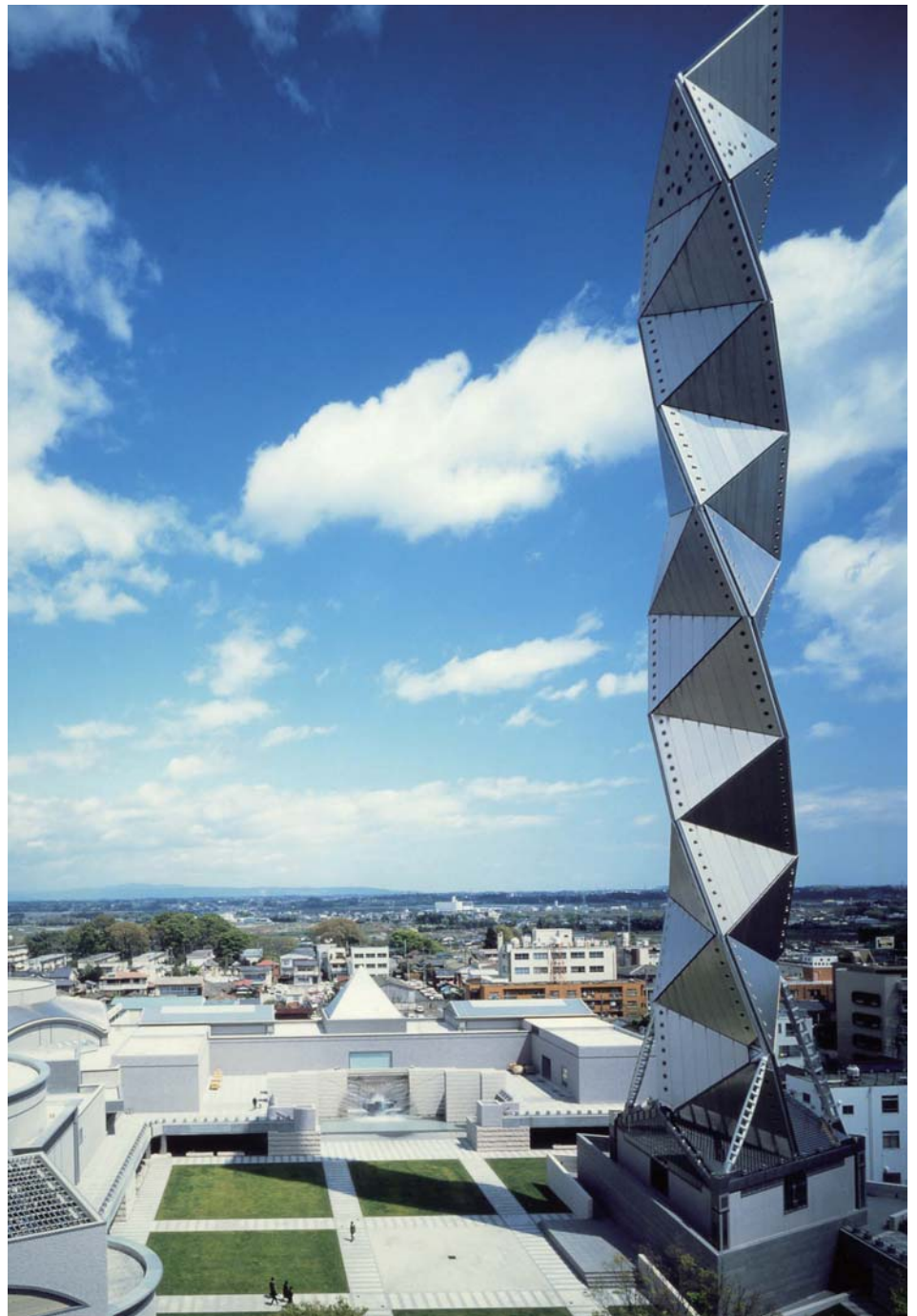
The Mito tower is constructed of almost 18 tons of First Grade titanium.
